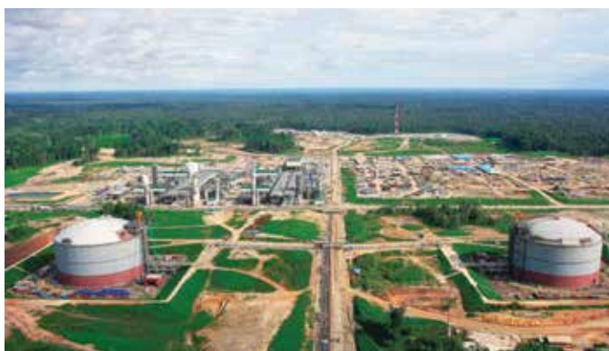
Production Facility - BP Tangguh
