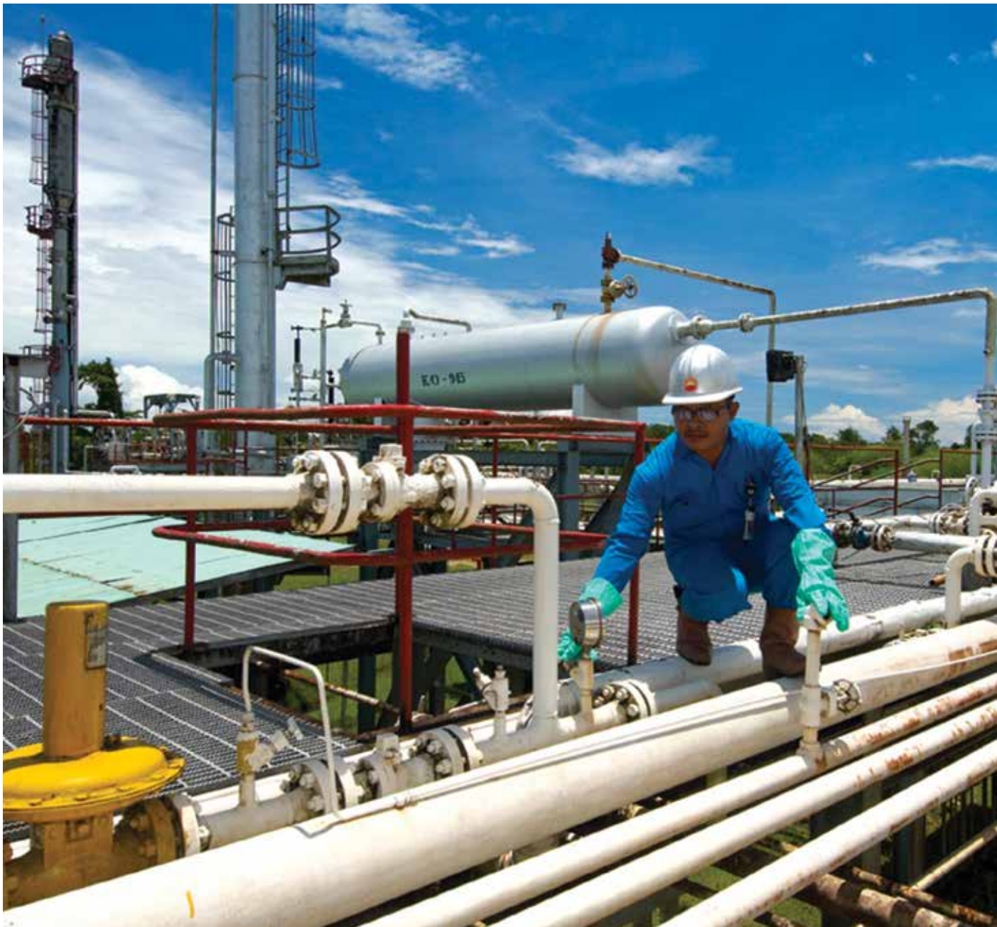
Production Facility - PetroChina
