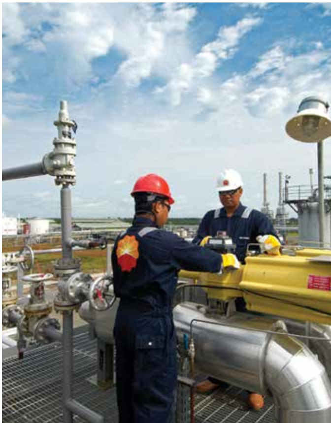
Production Facility - PetroChina
